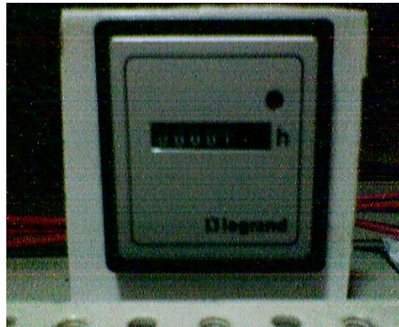
Figures 4 and 5: Monitoring Device Installed – kW-hr Meter & Run-hr Meter, York Air-Cooled System Model: YDAJ98MU7-50PA
