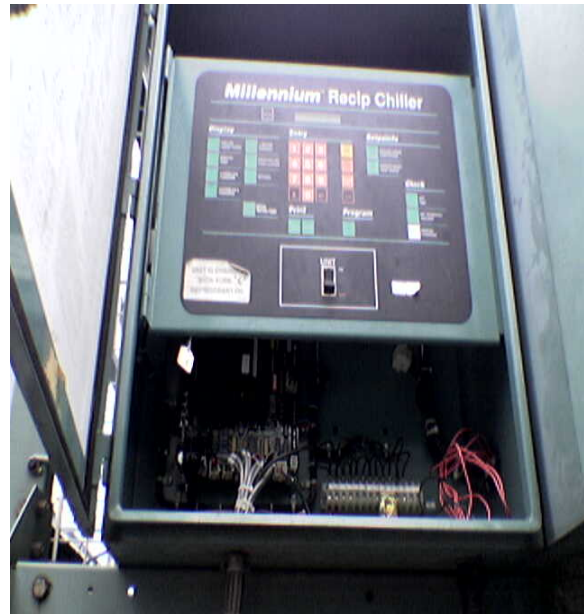
Figures 2 and 3: Far East Square Shopping Complex, Roof Top, Chiller No 3, York Air-Cooled System Model: YDAJ98MU7-50PA
